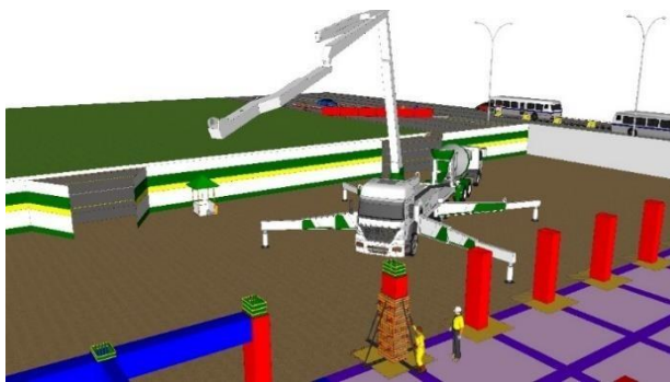
Figure 15. Column Casting Beam and Slab Work (Zhu et al., 2020)
