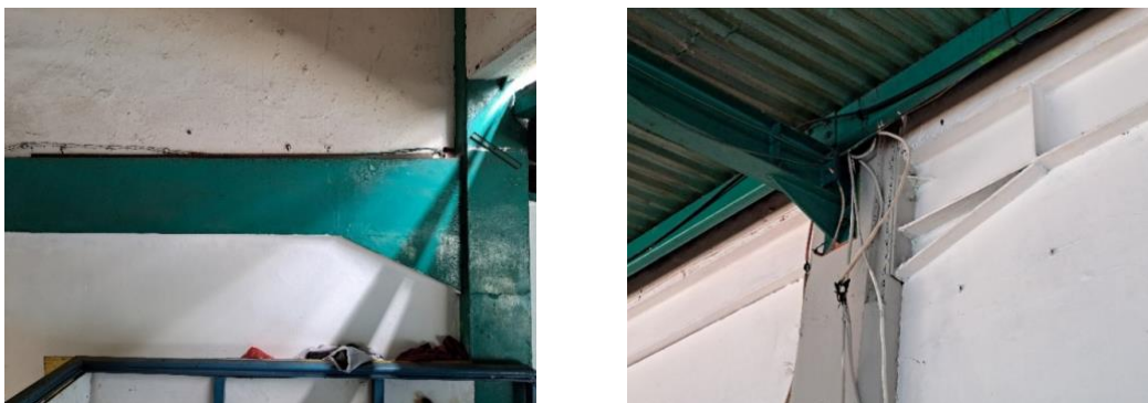
Figure 6. Existing Condition of Beam-Column Joint Connection
