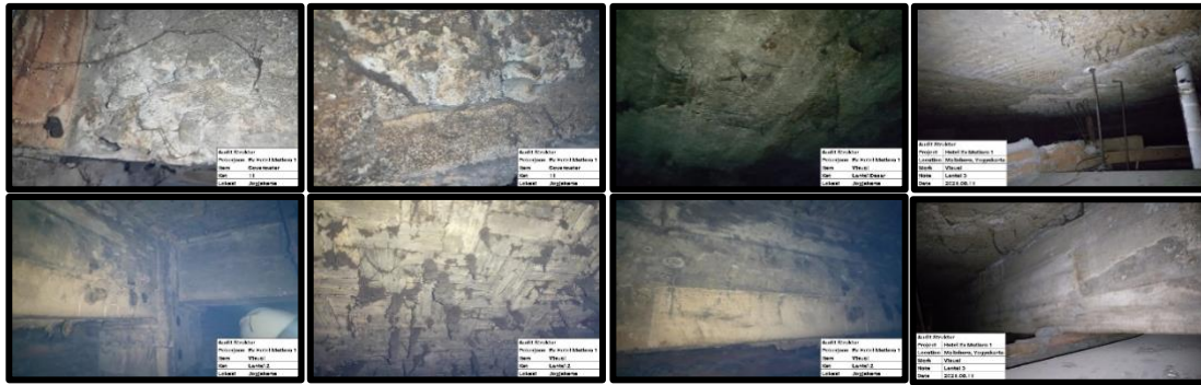
Figure 1. Existing Condition of Ex. Hotel Mutiara 1 Building
