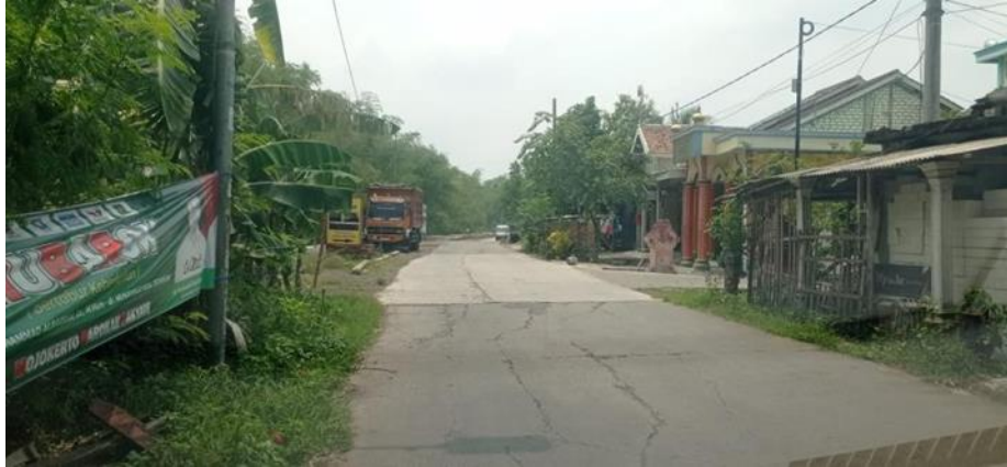
Figure 4. Corner Breaks
