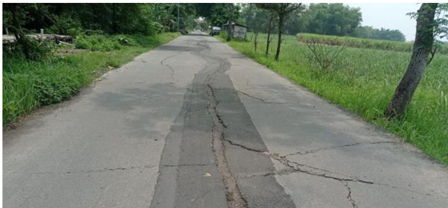
Figure 3. Joint Spalling
