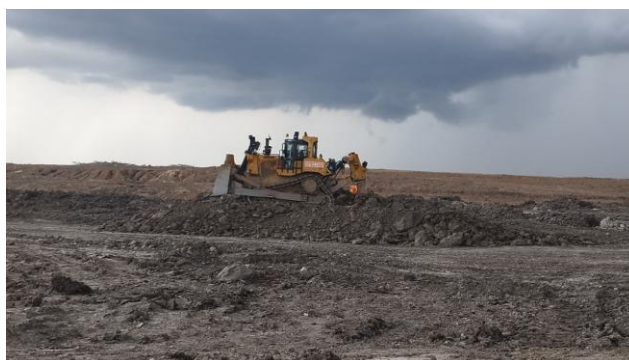
Figure 11. Construction of two-meters layer of waste dump
