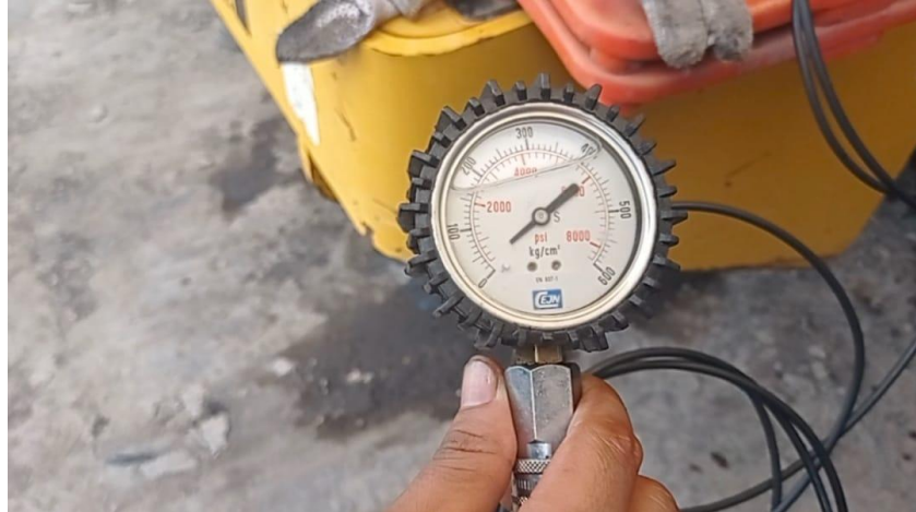
Figure 6. Process of checking hydraulic pressure using the Genuine Komatsu tools on the Sakai compactor unit after the coupler modification
